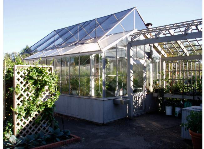
**Figure 6.** A hobby greenhouse with glass sidewalls and polycarbonate roof covering.
