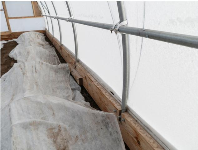
**Figure 5.** Baseboard installed at the base of a high tunnel to reduce cold air movement into the protected growing area. Note the polyethylene covering has been sealed tightly for winter, and the grower is using a fabric covering to keep lettuce warmer on the ground bed.
