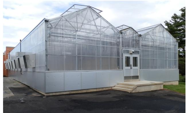
**Figure 7.** A large production greenhouse with corrugated polycarbonate covering and insulated curtain wall.
