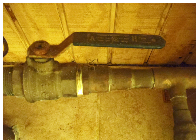
Figure 1. Shut-off valve for water line in the open position.
