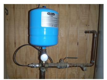
Figure 2. Small pressure tank associated with a VFD-controlled water pump.
