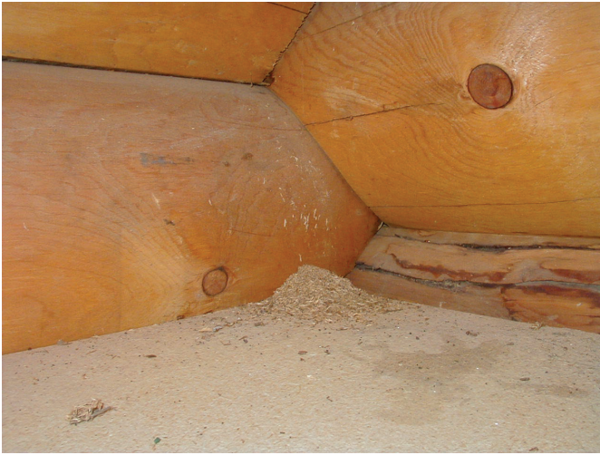
Figure 7. Typical pile of saw dust discarded from carpenter ant tunneling. Saw dust won't be seen inside wall voids and other inaccessible locations. (Photo credit: Barbara Ogg).
