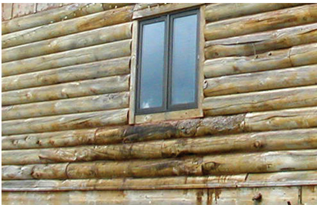
Figure 5. Rotted wood under the window of a log home. (Photo credit: Barbara Ogg).
