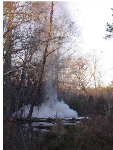
Figure 10. Use of explosives to remove a beaver dam and reduce flooding (Photo by Michael T. Mengak).
