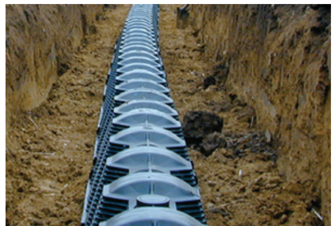
Figure 3. Drainfield with chamber prior to backfilling with soil for a gravelless system.
