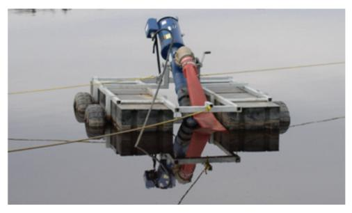
Figure 4. Floating pump installation for pumping lagoon water to a center pivot.
