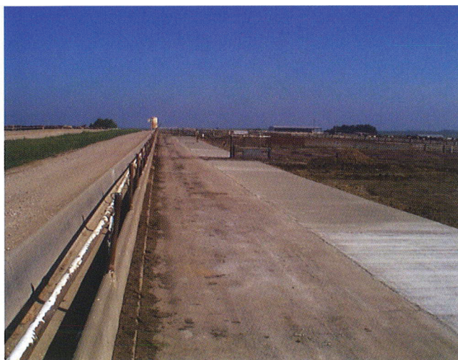
Figure 10. Bunkline and apron layout. Note that the pad has been extended, and that while the waterer is located in the centerline, it is not far enough from the bunks.
