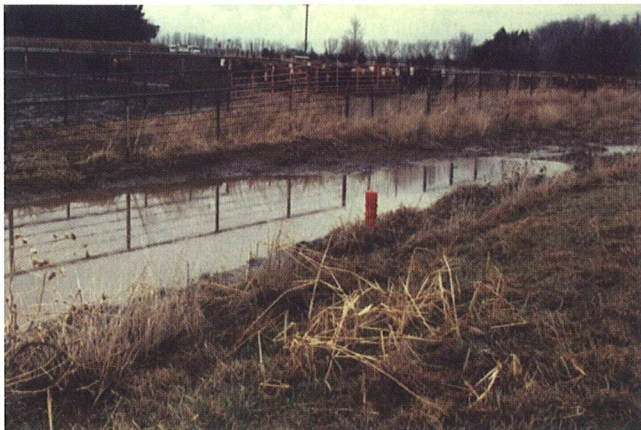
Figure 14. A debris basin collects runoff and slowly releases liquids so that solids settle and dry for easy clean out.
