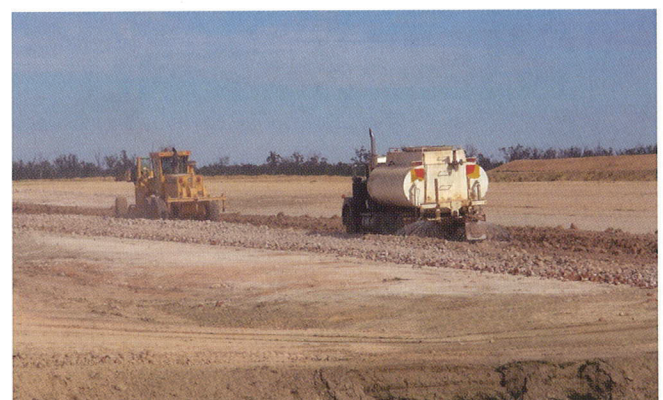
Figure 5. Water addition and wheel tire compaction of feedlot pad (pen surface).
