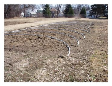
**Figure 15.** Assembled hoops located near ground posts ready to be tilted into position.
