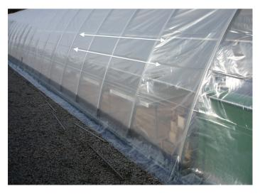
**Figure 17.** Positioning of polyethylene is simply done by aligning gusset creases with wall purlins.
