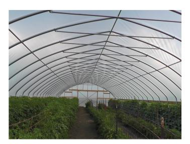
**Figure 11.** Cross bracing was installed in the peak of this high tunnel to stabilize the structure during high winds, heavy rains, and snowfall.
