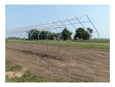
**Figure 9.** Creating a level site through cut and fill excavation will result in compacted soils that are unlikely to be suitable for in-ground plant production.
