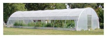
**Figure 5.** Roll-up sidewall components provide options for improved interior temperature management. Note overlapping wall blanks at both ends of the roll-up wall to prevent cold air infiltration.
