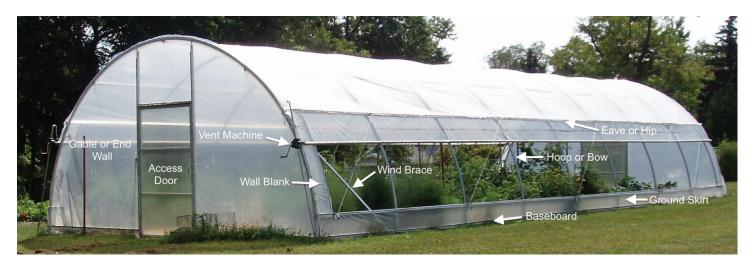
Figure 1. Common high tunnel terminology.
