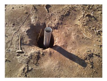
**Figure 14.** To create a pier foundation for the hoops, holes are drilled into the soil and filled with concrete around the ground posts.
