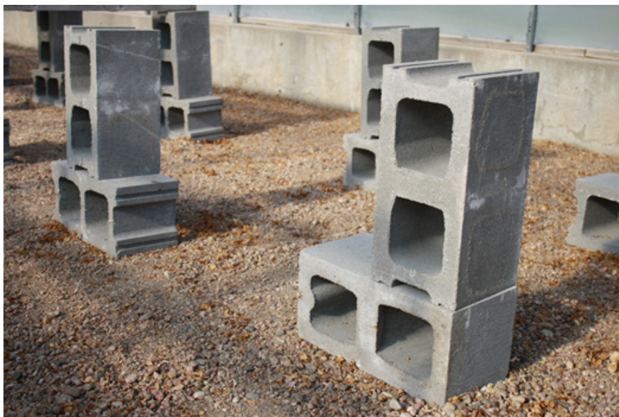
Figure 1. Blocks set in position on a level floor. Note end blocks held flush with terminating end of bench and “in line” blocks are centered for stability.
