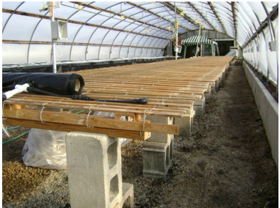
Figure 3. Completed block and fence bench. Note: bench fabric (fence) is centered on support members with 1 foot extending on either side and held taut by deck screws installed at each end.
