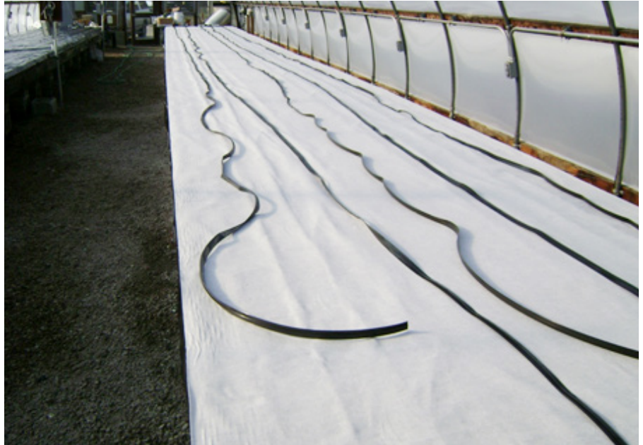
Figure 5. Seep hose is laid in rows roughly 14 inches apart for uniform distribution of water across the entire capillary mat surface and connected to water supply using fittings supplied by the CapMat II™ Distribution Kit.
