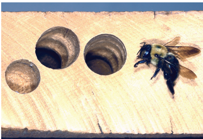
Figure 19. Carpenter bee holes in the exposed end of a floor joist.
