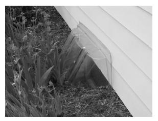
Figure 10. Window well cover. Photo by Stephen M. Vantassel.
