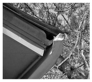
Figure 2. Tree squirrel hole in a soffit. Photo by Stephen M. Vantassel.
