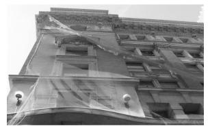
Figure 8. Nets must be maintained to prevent bird access to sensitive areas. Photo by Stephen M.Vantassel.
