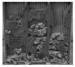
Figure 4. Insulation that has been damaged by house mice. Photo by Robert M. Timm.
