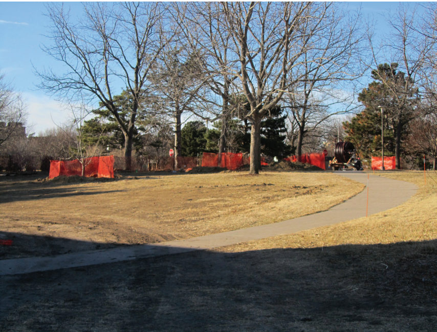
Figure 5. The simplest way to protect the root zone from equipment damage and inadvertent changes in grade during construction is to install substantial fencing — and enforce this barrier with diligent observation.
