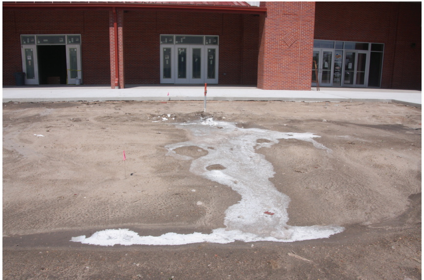
Figure 6. The best protection from damage by foreign substances is to keep spills from happening. Removal of contaminated soil may be the only option if remediation is necessary.
