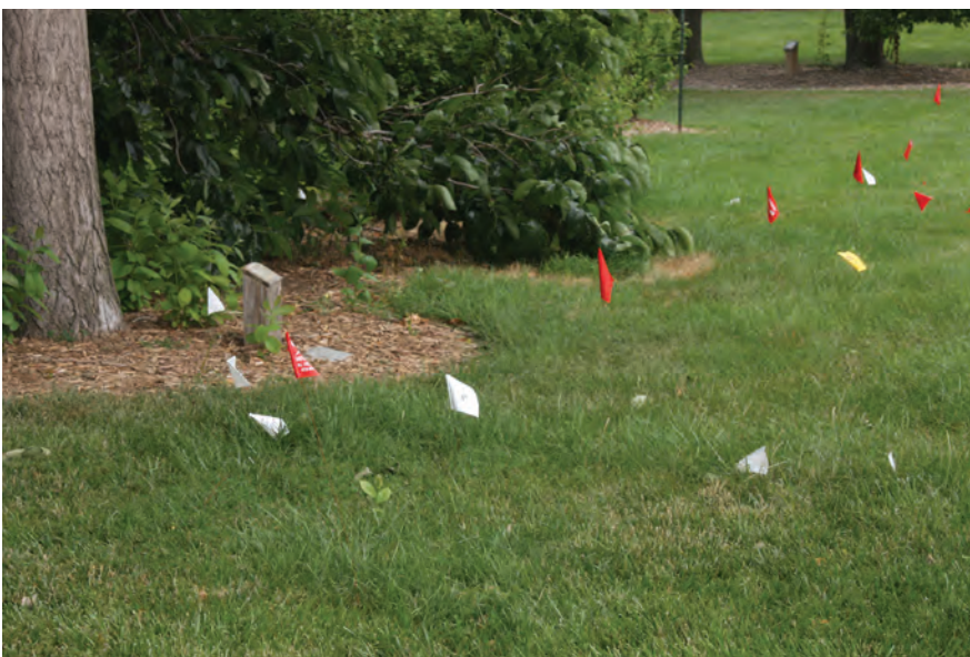
Figure 1. Mark all private utilities and lines prior to finalizing the locations of landscape beds and individual plants.
