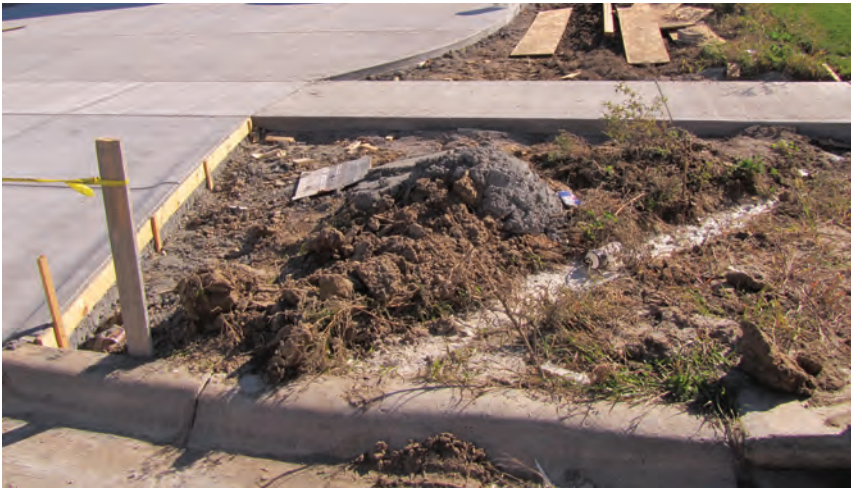
Figure 4. Plant roots may be unable to penetrate the barrier created by compacted soil, resulting in shallow surface roots and a reduced ability to survive drought.
