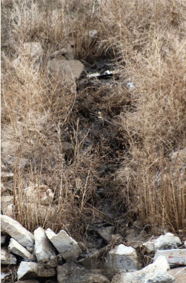
**Figure 9. Erosion of lagoon berm from broken discharge pipe. (Photo credit: Jill Heemstra)**
