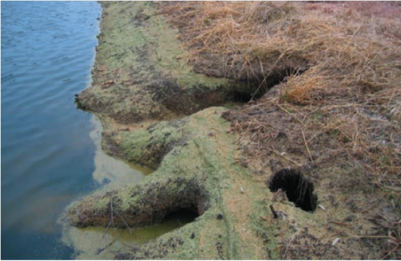
**Figure 6. Erosion or animal burrowing on berm of lagoon. (Photo credit: Powell, et al., 2005)**
