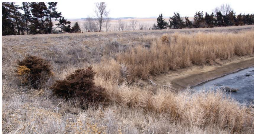
Figure 5. Excessive vegetation growth on the inside berm of a lagoon. (Photo credit: Jill Heemstra)
