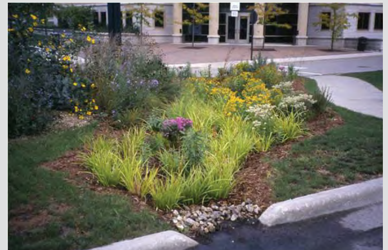
This rain garden collects runoff from the street.
