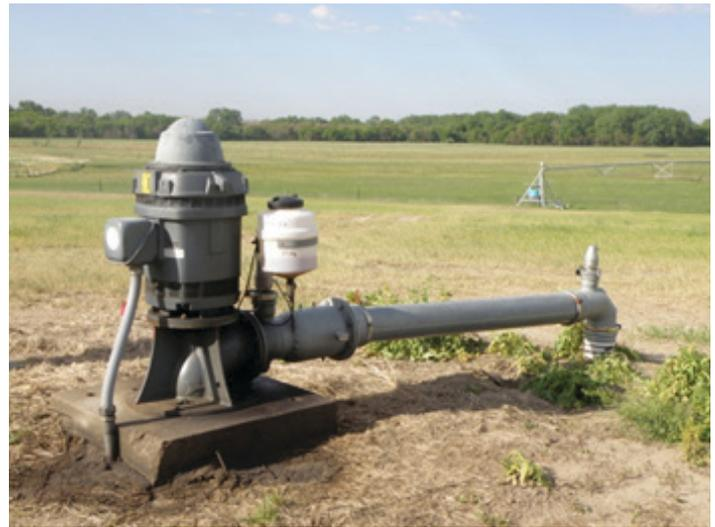
Figure 79. Electric motor for pumping irrigation water.
