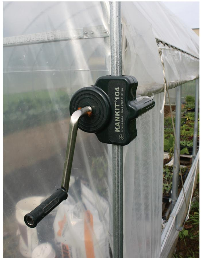
**Figure 6.** Hand crank roll-up window vent machine
