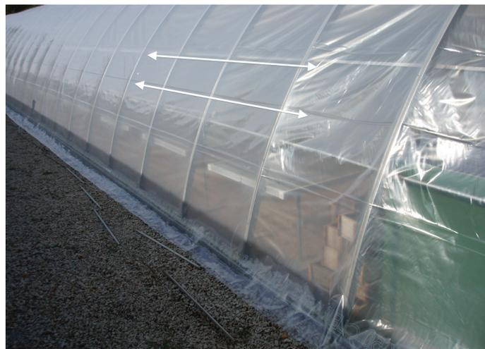
**Figure 17.** Positioning of polyethylene is simply done by aligning gusset creases with wall purlins.
