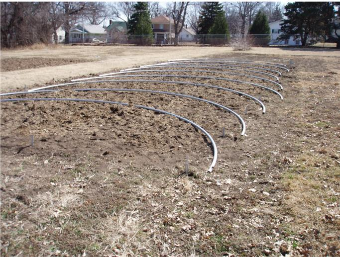
**Figure 15.** Assembled hoops located near ground posts ready to be tilted into position.
