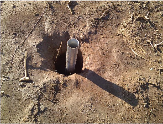
**Figure 14.** To create a pier foundation for the hoops, holes are drilled into the soil and filled with concrete around the ground posts.
