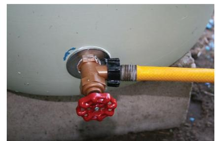
Figure 4. Rain barrel water outlet — a hose bibb with hose attached for dispersing water.
