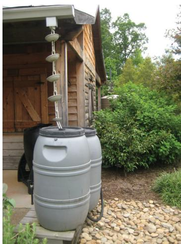
**Figure 1.** Rain barrel using a rain chain in place of a downspout.
