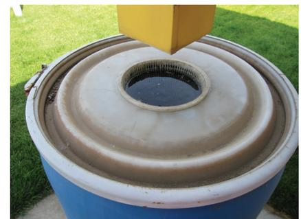
Figure 3. Barrel placed beneath the downspout. Excess water may overflow more readily out of this type of opening.
