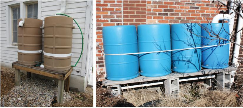
**Figure 6.** (Left) Barrels securely elevated and anchored with a sturdy platform, straps, and connection to the building for safety. (Right) Barrels poorly supported on wood planks and concrete blocks and tied with a single rope around all barrels. This is not as strong or secure as using a single strap on each barrel.
