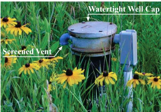
Figure 3. A watertight, secure cover caps the top of the well.
